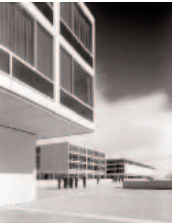
ABOVE: U.S. Air Force Academy, Colorado Springs, Colorado, from the exhibition Building Images .
