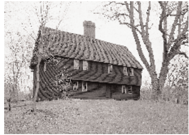
LEFT: Capen House, Topsfield, Massachusetts.
