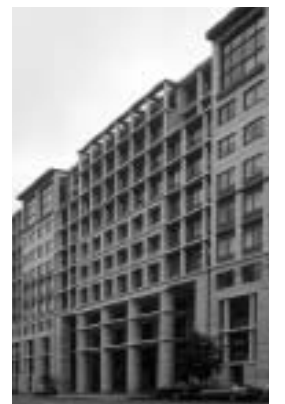
top / AFL-CIO Headquarters, Washington, DC, 1954, a commercial building based on the open, rational concrete frame, here obscured by a façade with separate door and window openings.
