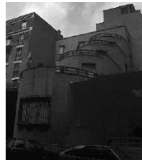
top / Siège Social de la Société Hennebique, Paris. The evolution of building and zoning codes in Paris reinforced the stone masonry culture. Internal cast iron frames could not be revealed at the first three floors; cladding had to be in stone. This building obeys the 1902 code, which required sculptural relief on façades.
