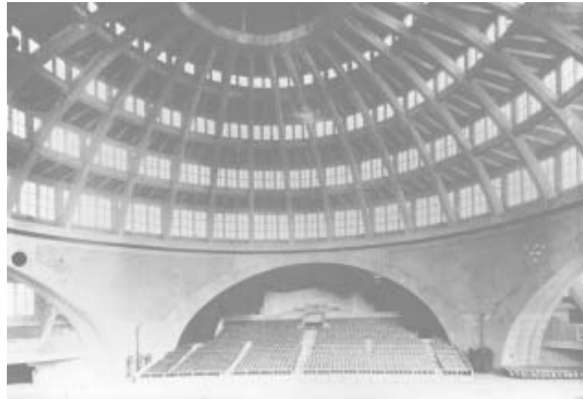
above / Jahrhunderthalle (Centenary Hall), in what is now Wrocław, Poland, by Max Berg, featuring a ribbed concrete dome and clerestory windows. Photograph courtesy of Dr. Jerzy Ilkosz, Director, The Museum of Architecture in Wrocław
