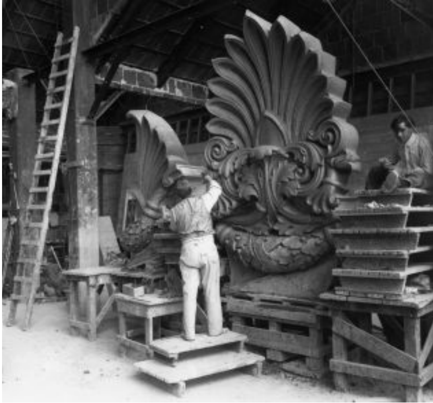
above / A sculptor working on a terra cotta acroterion in the Northwestern Terra Cotta Company shop, Chicago, 1914. Gift of Edward J. Mertes; Northwestern Terra Cotta Collection; Collection of the National Building Museum.
